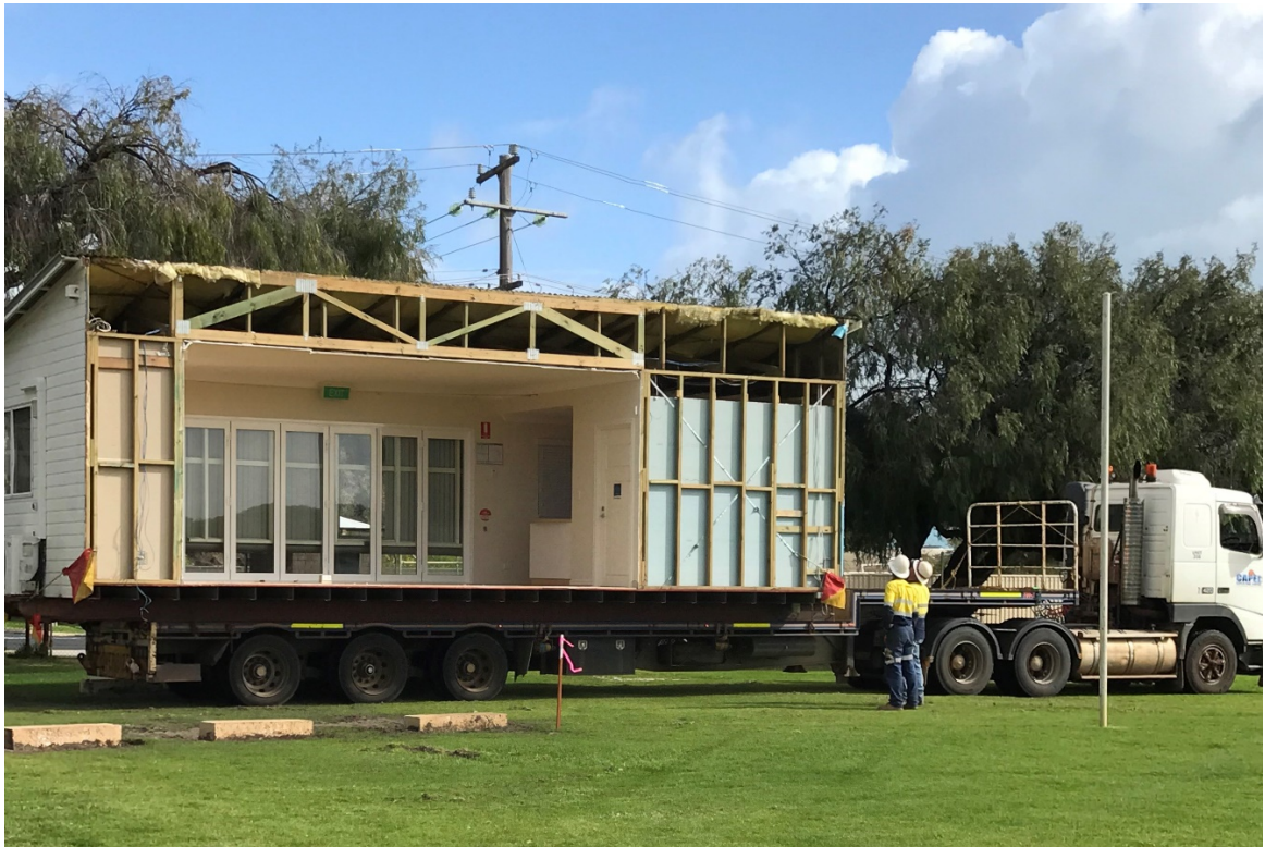
In with the New (First Half)
